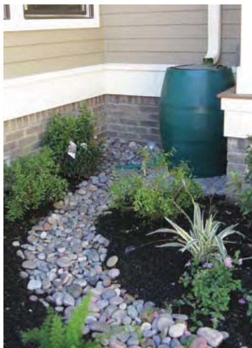
Rainwater collection systems are an integral part of sustainable designs.
